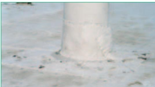
Sealed pipe penetration with BENTOFIX®
