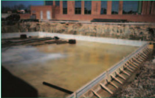
**BENTOFIX® BFG 5000** is manufactured in three standard sizes and is delivered in rolls. Depending on the particular application, the choice of roll size allows simple on-site storage and handling. Full waterproof seals are achieved by simple overlapping, making installation quick and easy. The dimensions of the liners are as follows
