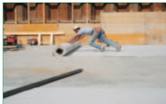
In a dry state, **BENTOFIX® BFG 5000** has a thickness of 6 mm. Once hydrated, the thickness of the product increases by approx. 4 to 5 mm after a few days of free swelling (not subjected to any confining stresses from external sources). Providing the product remains hydrated, this value does not vary over time.
