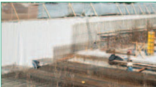
Steel reinforcement being placed in front of BENTOFIX®
