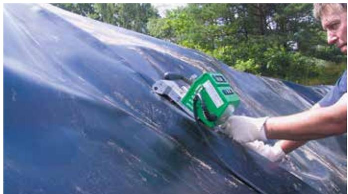
Non woven geotextiles and geomembranes used for sealing of water reservoirs
