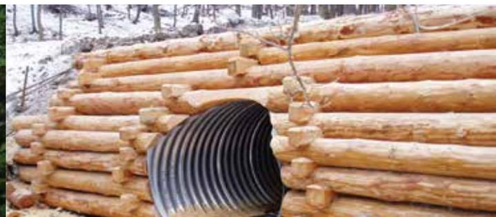
Helically corrugated steel pipes HelCor® and pipe-arches HelCor PA used as culverts and animal underpasses
