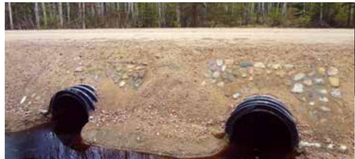
Culverts and underpasses for animals made of high density polyethylene PECOR OPTIMA® pipes and polypropylene Pecor Quattro pipes
