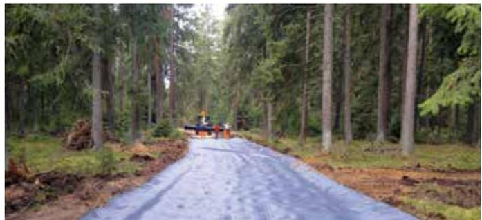
Woven and non woven for reinforcement and separation of low-bearing soils
