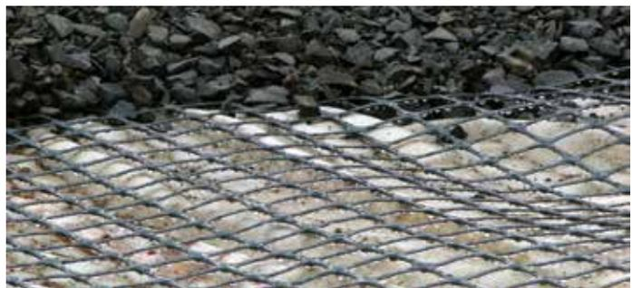
Geogrids for soil stabilization and reinforcement
