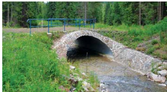
Flexible steel structures MultiPlate MP200 and SuperCor® used as culverts, bridges and animal under and overpasses
